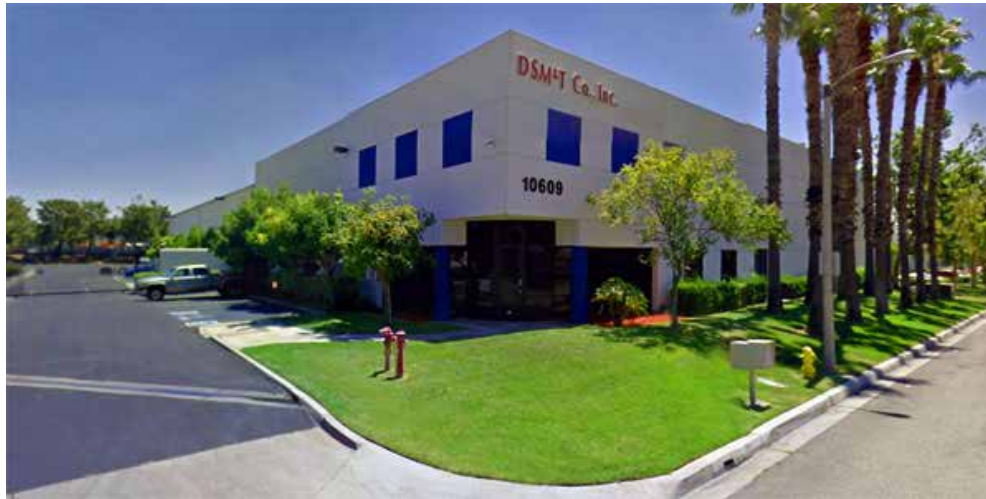
Headquarters and Main Manufacturing Facility. Fontana, CA, USA
